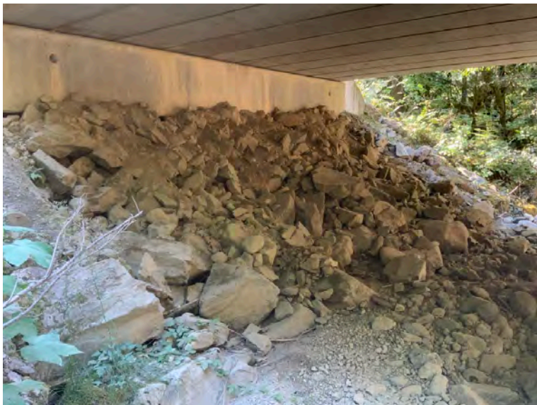
Left Bank Abutment when facing downstream
