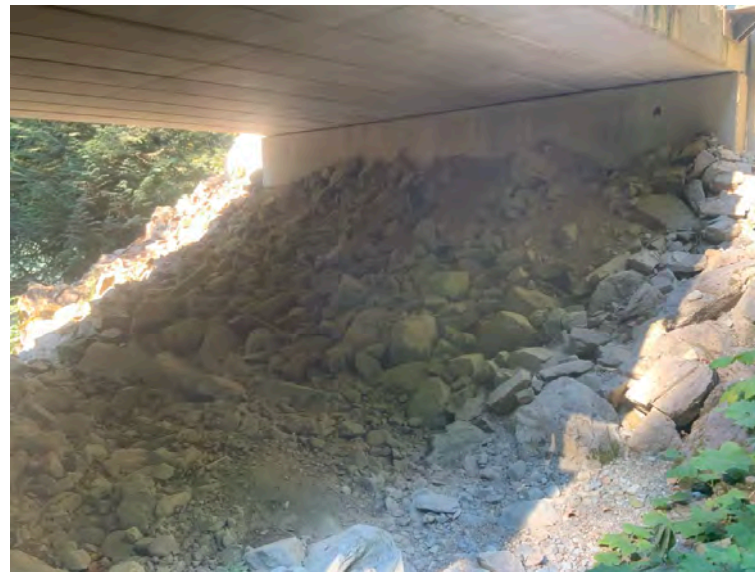
Right Bank Abutment when facing downstream
